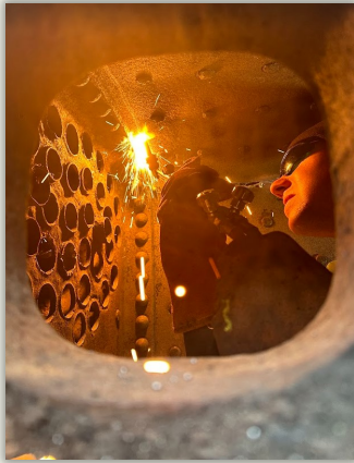
Cutting out the Crown Sheet
