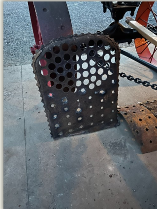
Firebox Sheets Removed
